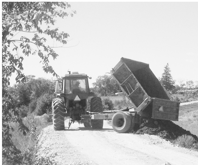
Wood chips (top left) take nitrates out of the water. Top right, soil is dumped on a berm constructed to divert runoff.
