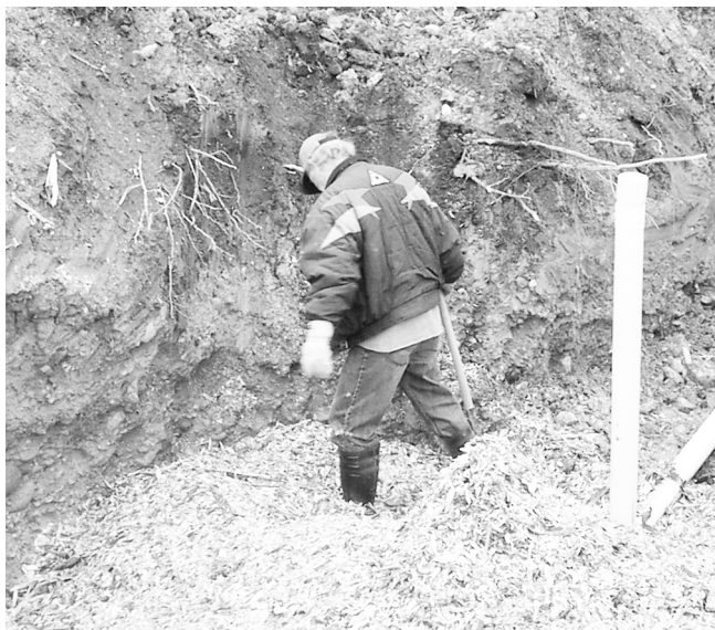
Wood chips (top left) take nitrates out of the water. Top right, soil is dumped on a berm constructed to divert runoff.
