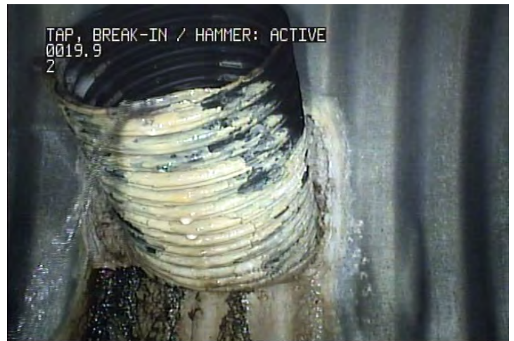
TBA - Tap, Break-in / Hammer: Active @ 19.9 m.
