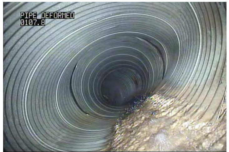
D - Pipe Deformed @ 107.8 m.
