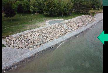
Properly designed sloping stone structures are recommended over vertical walls for glacial till shorelines
