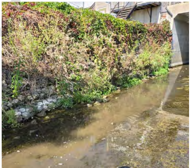
Gabion basket wall, west side just south of conduit
