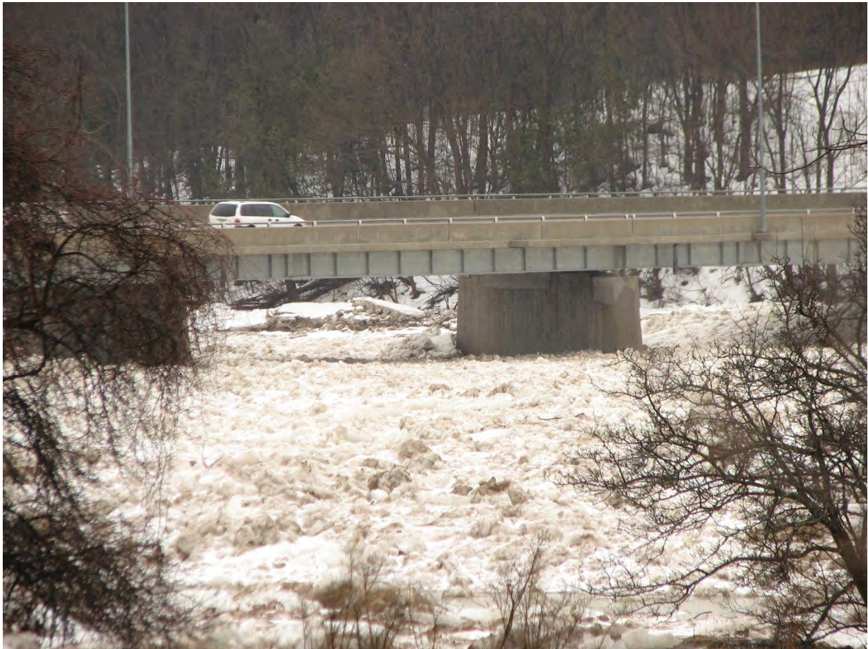
Figure 3. Ice building up at the Highway 21 bridge during an ice jam event in 2011
