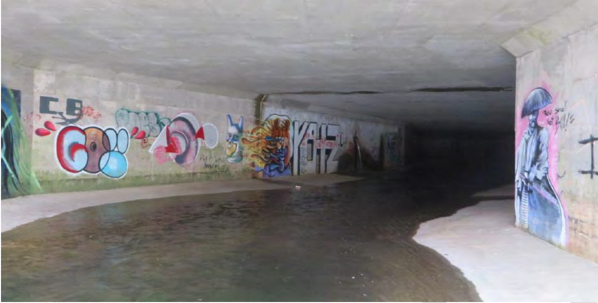
Inside of conduit, looking south
