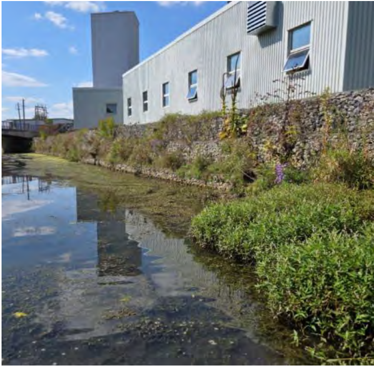
Gabion Basket Wall, west side north of Union St.
