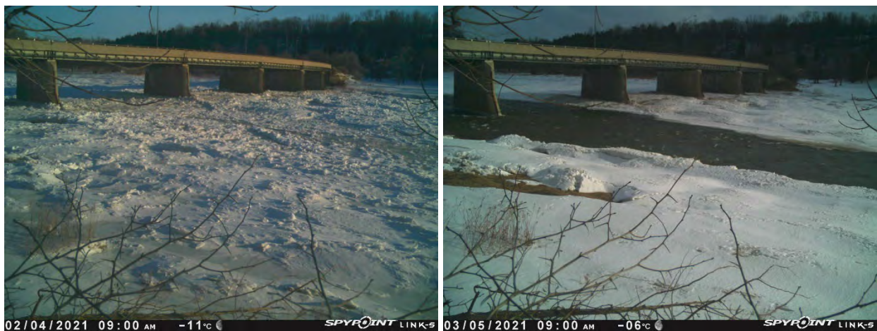
Figure 9. Sample photographs from Saltford setup: near complete sheet ice cover (left); flowpath eroded through ice after thaw (right)
