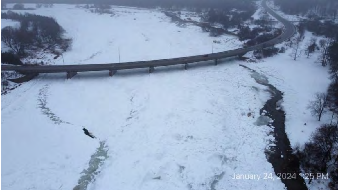
Figure 5. Photograph taken with use of a drone, easily identifies flow pathways and weakened sections of ice cover
