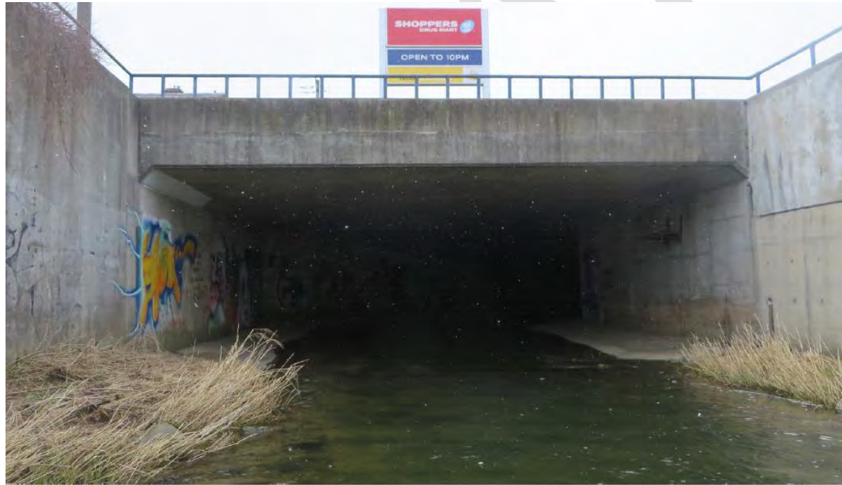
North Entrance to the Conduit, looking south
