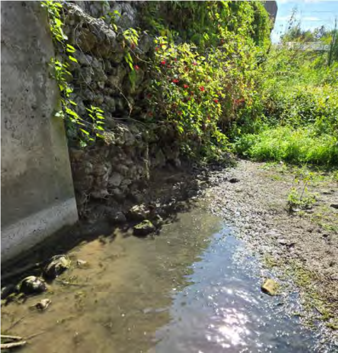
Gabion Basket, east side just south of conduit
