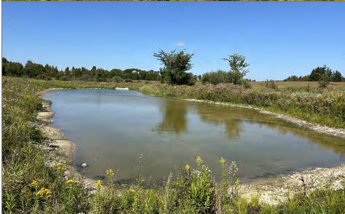
Settling ponds help keep sediment from reaching the river.
