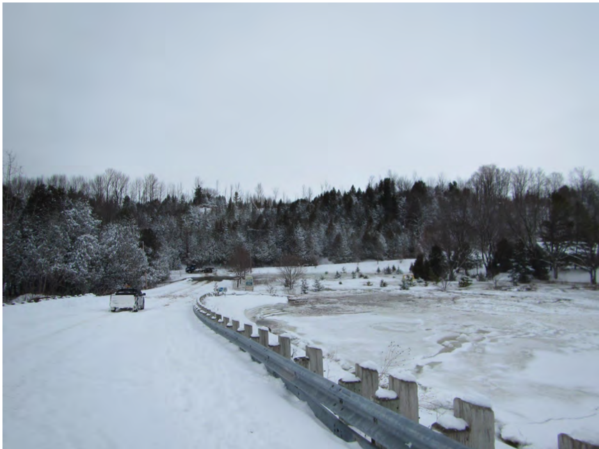
Flood waters spilling into the Parking lot north of the Fishway in 2016
