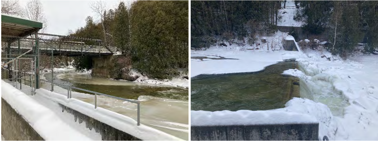
Figure 4. Port Albert fishway (left); concrete drop structure and turbulent water (right)
