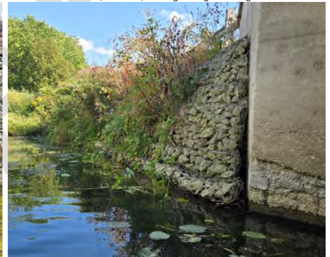
Gabion Basket Wall, east side north of Union St.
