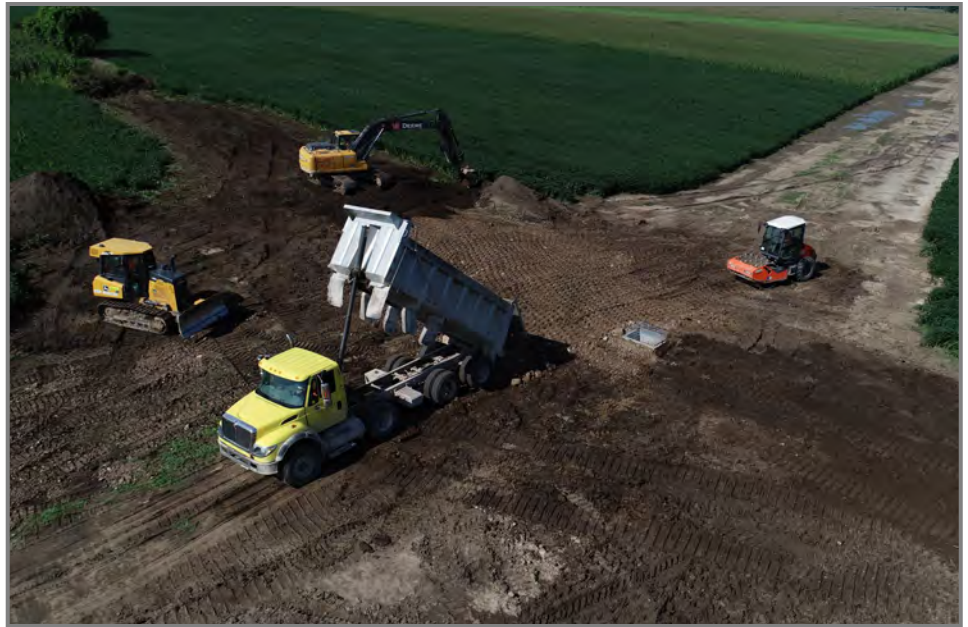
Aerial photos taken in the Garvey-Glen watershed show how construction of berms and grassed waterways keep water off the fields during rainstorms which protects the soil and keeps the water clean before it ends up in Lake Huron.
