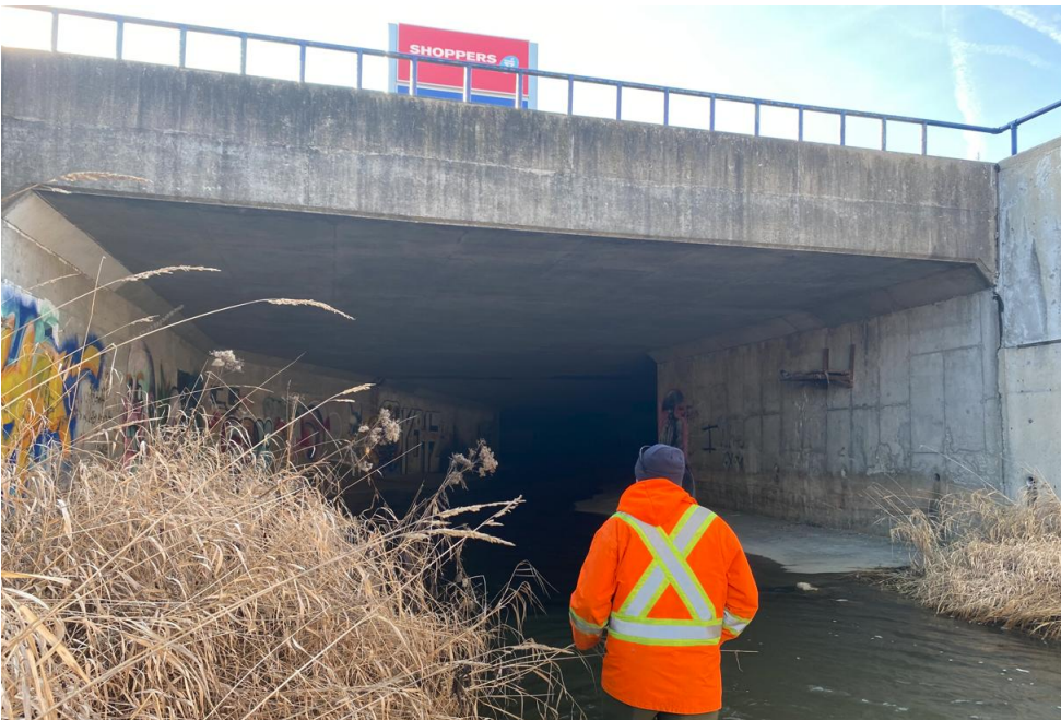
Figure 2: Listowel Conduit, under main street
