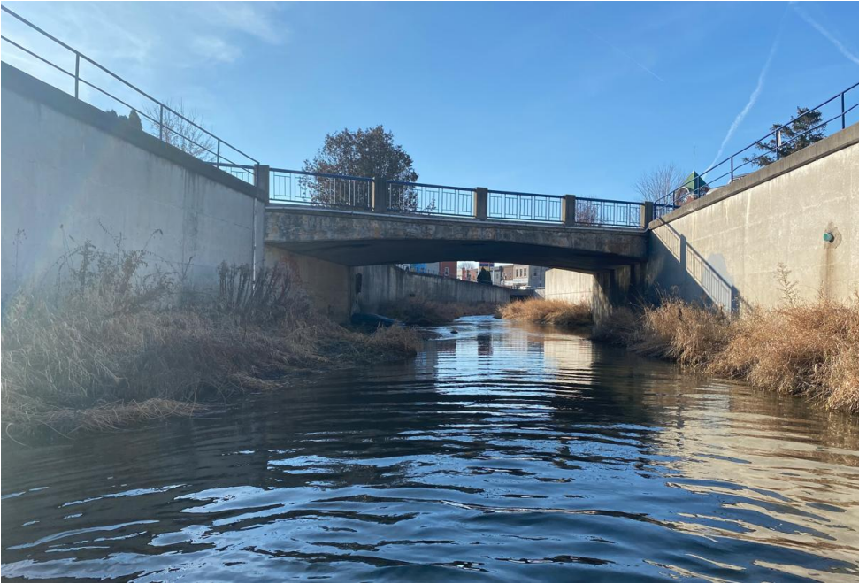
Figure 1: Listowel Conduit, retention walls
